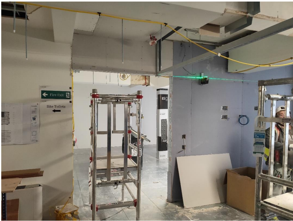
Level 3 Offices Bulkheads and Partitions
