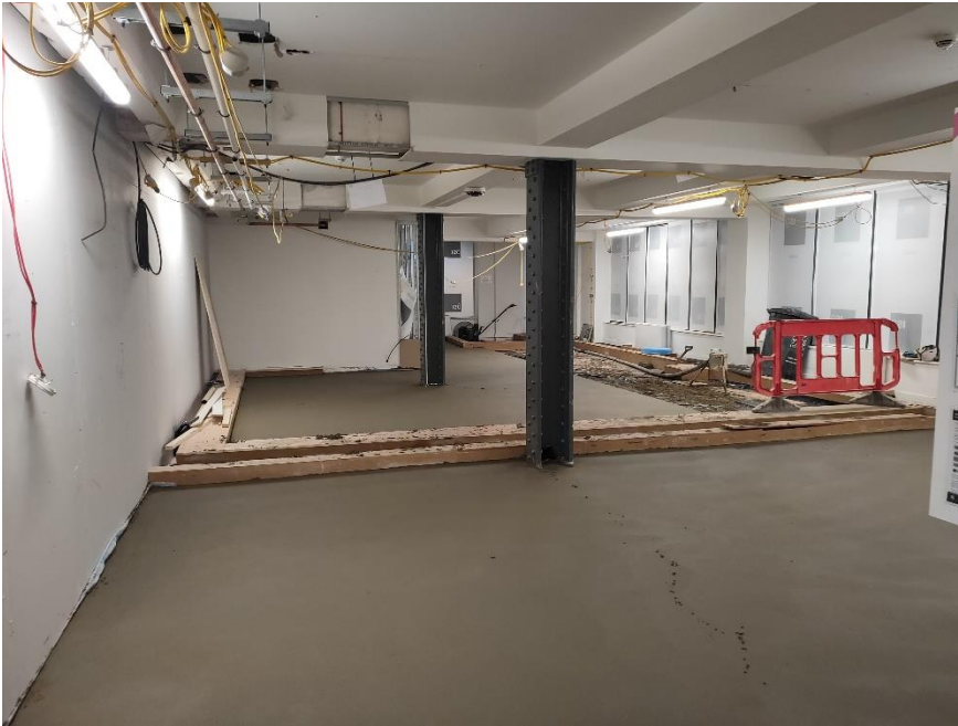
Basement Gym Floor Screeding
