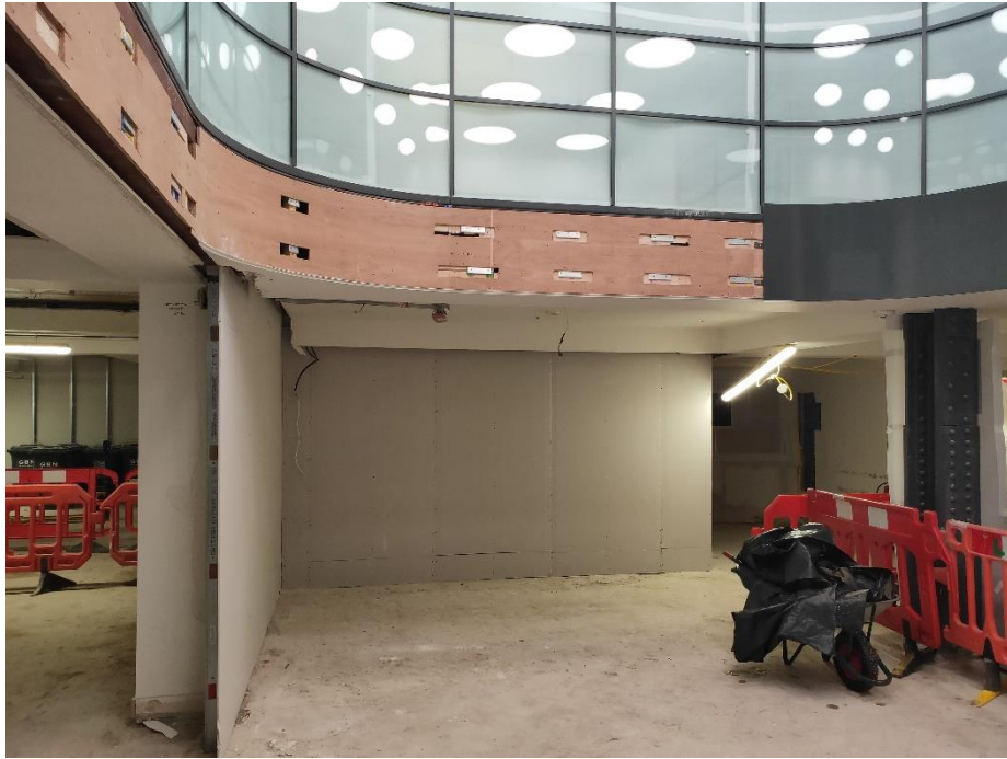
Ground Floor Reception Partition Formation
