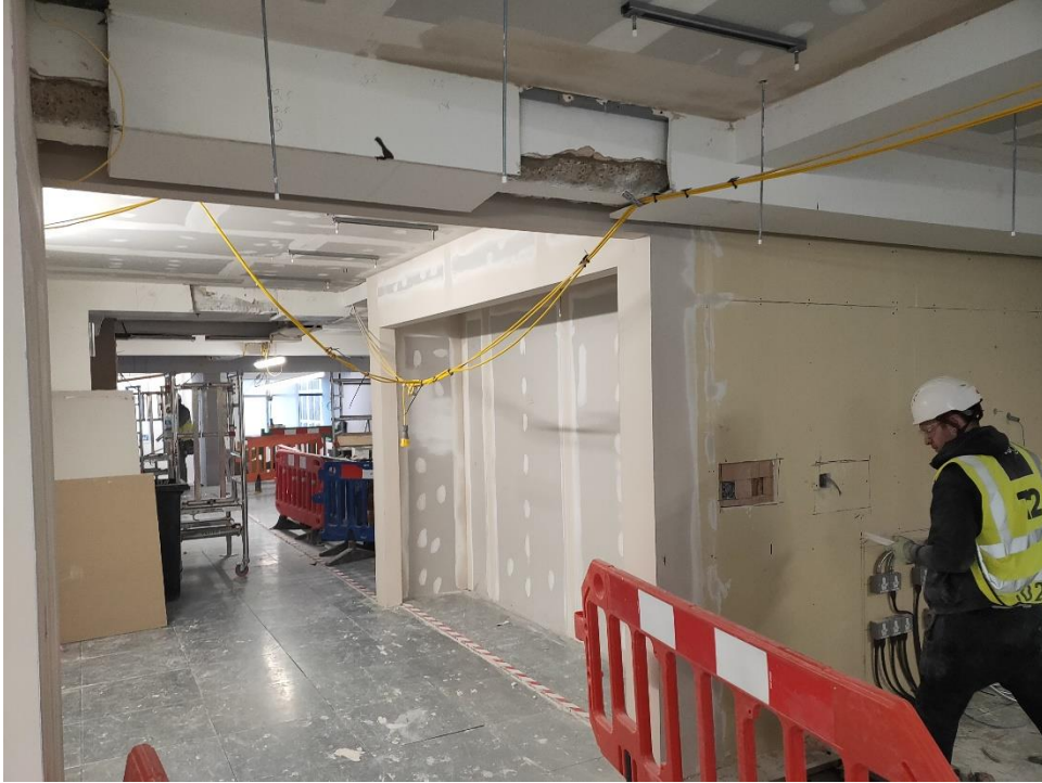
Level 5 Cloak Room and Arrival Space (taken from Café Area)
