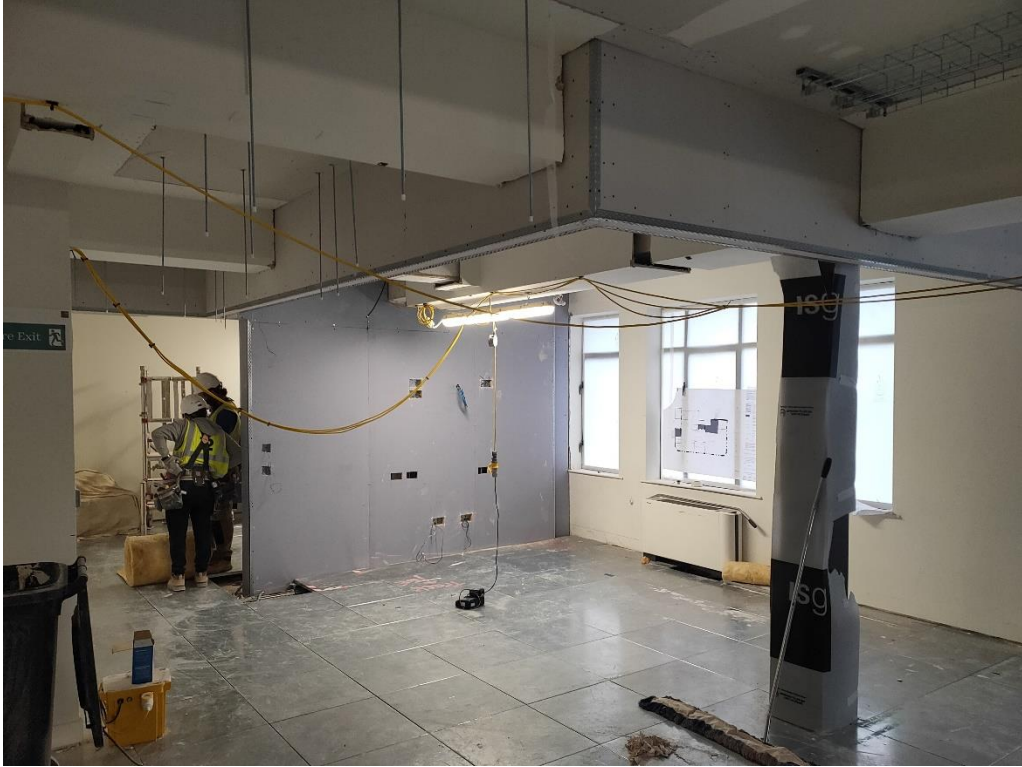
Level 4 East Offices (04.09 & 04.07)
